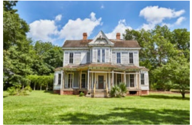
The Foster-Thomason-Miller House was first project of the Madison-Morgan Conservancy's Endangered Properties Revolving Fund. In 2019, the house was saved and sold to a conservation buyer. In 2018, the house was named as a "Place in Peril" by the Georgia Trust for Historic Preservation. Credit: Tony Clark, via Madison-Morgan Conservancy
