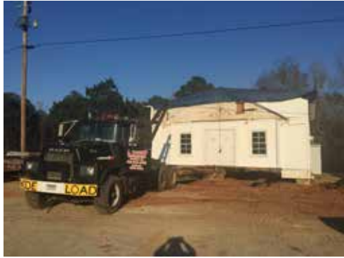
Before exterior with top off; getting ready to move to new site.
